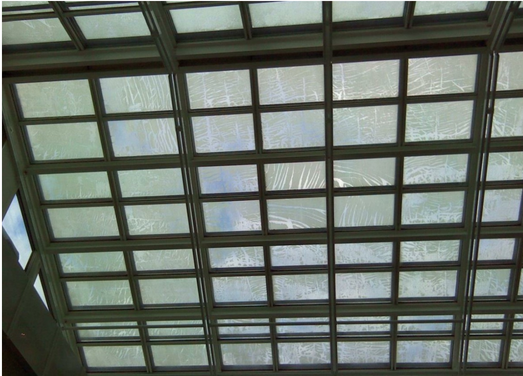
IATA's skylight before refurbishment
